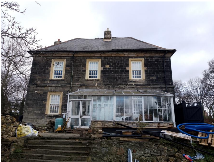
Figure 4: View of the surveyed building from the rear.
