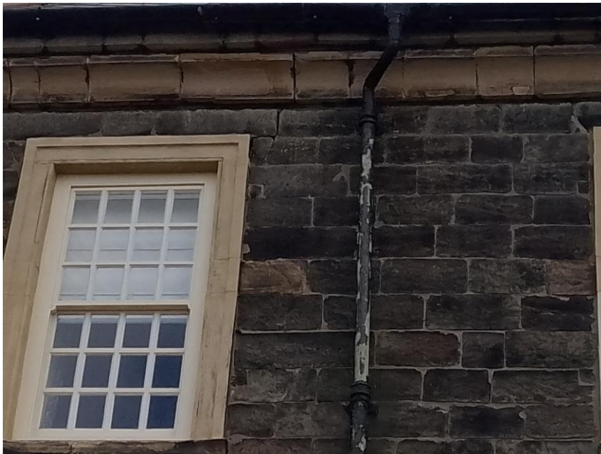
Figure 6: External walls with crevices suitable for bats.
