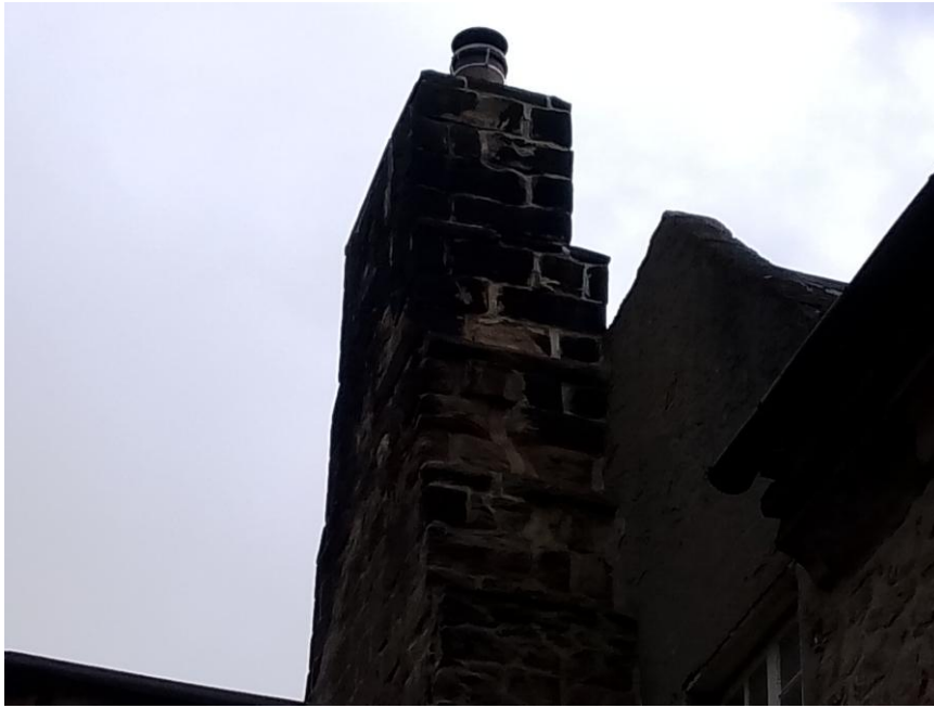
Figure 7: Close up of the chimney.
