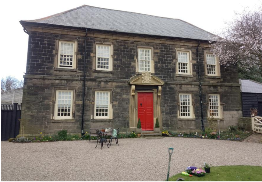
Figure 3: View of the surveyed building from the front.
