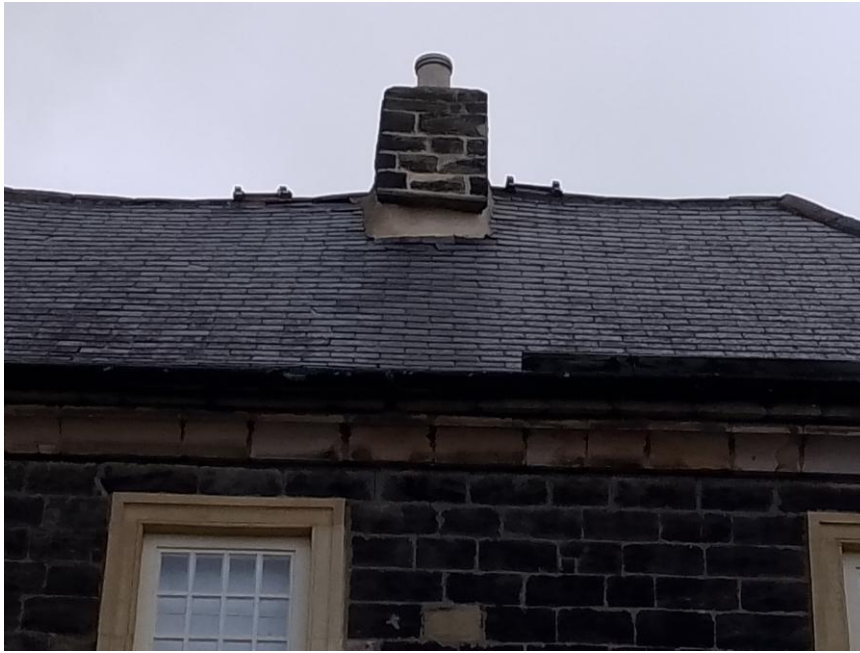
Figure 5: Close-up of the roof tiles and chimney.
