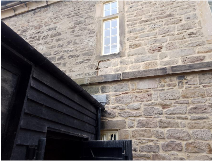
Figure 9: View of external stone walls.
